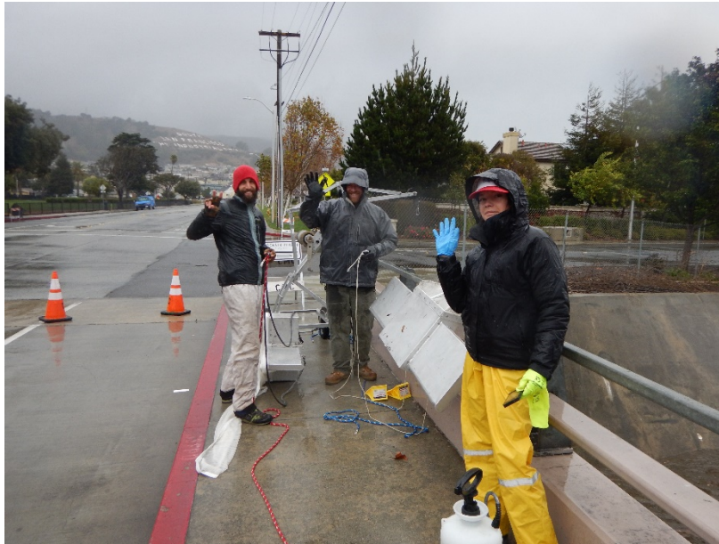
Figure 18. Traffic control measures at Colma Creek (cones and signage)
